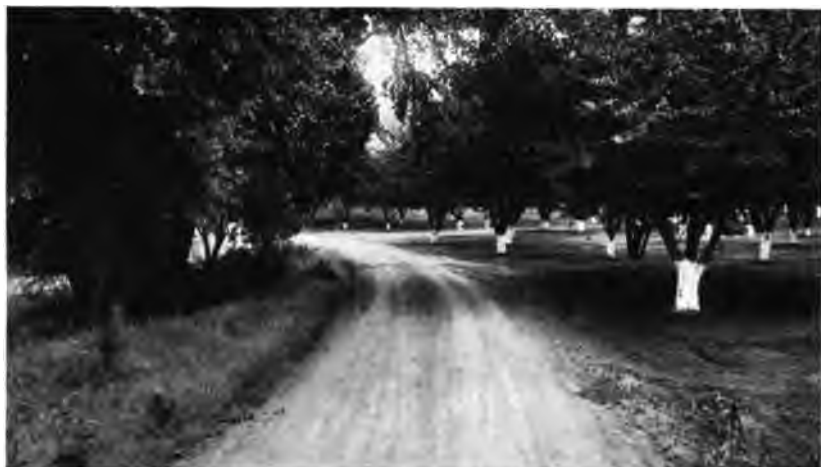
A neighborhood road of oil macadam in the orchard section
